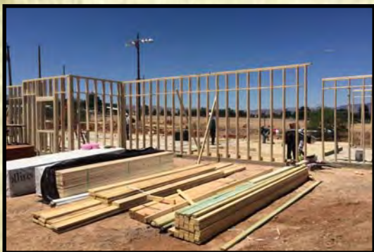
Central Arizona Lodge No. 14 's new building is bring framed
